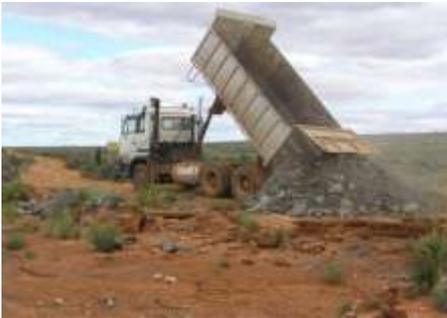
A 15T load of rock fill at the washed out boundary gate.
